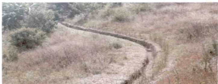
Contour ditch with newly planted soil-retaining grass barrier
