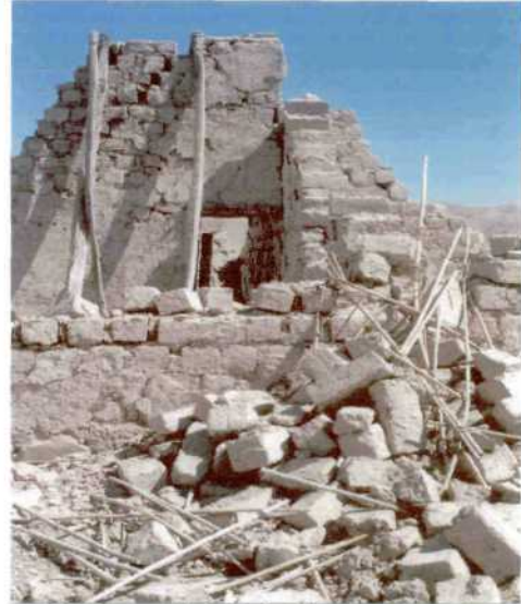
Destroyed house in Coplay, Moquegua
