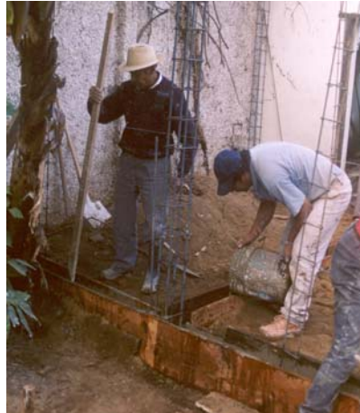
Pouring foundation footings
