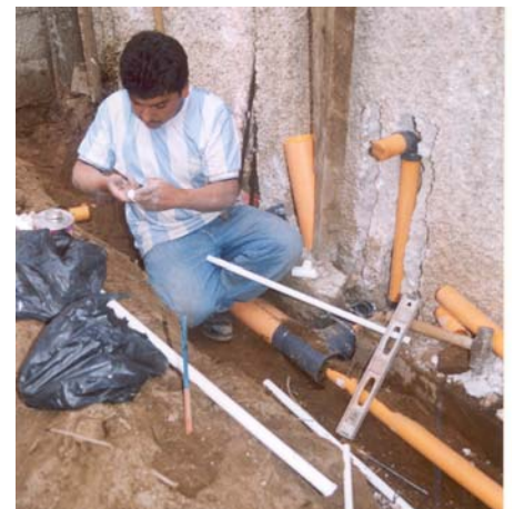
Plumbing the new bathroom
