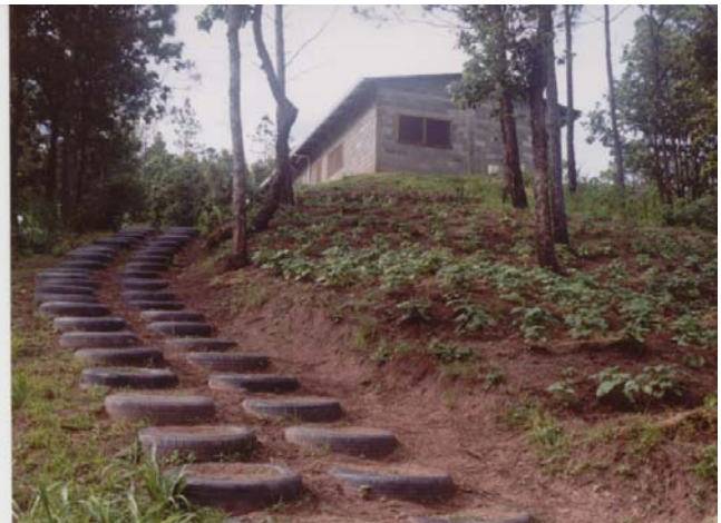
The creative use of resources is integral to Loma Linda's work in sustainable agriculture. Discarded tires are used to make steps up to the dorms.
